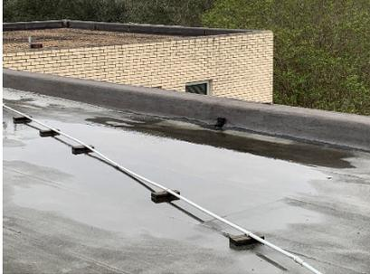
Water ponding on roof near drain
